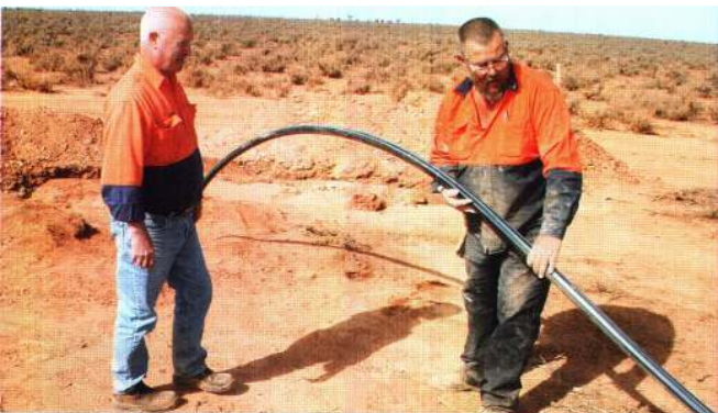
Russel Bluck and Mike Moore at a backfill site
