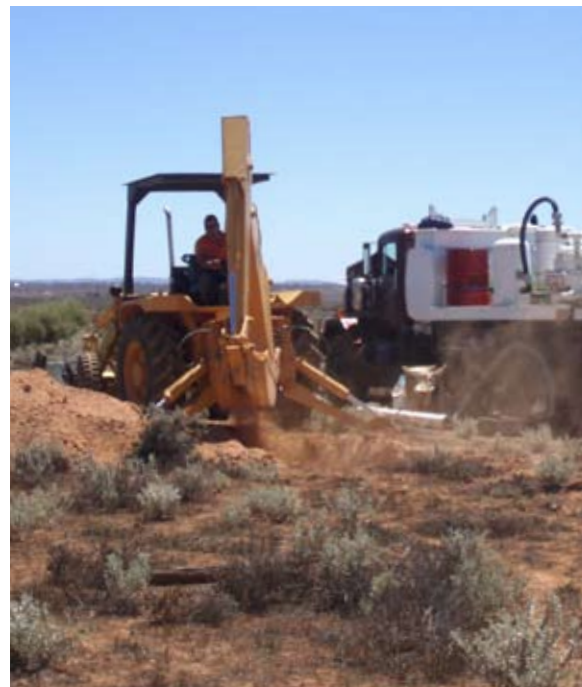
Drill site preparation for rotary mud drilling; Muckanippie
