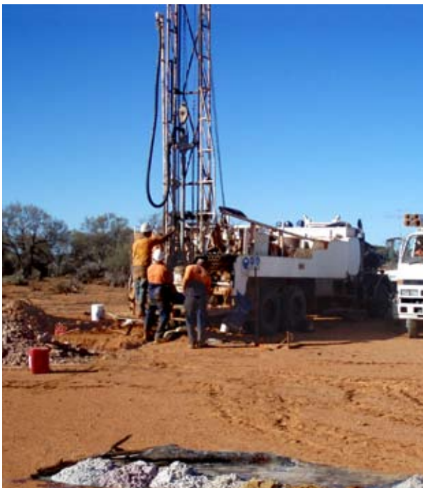
Rotary mud drilling operations; Kingoonya Palaeodrainage System
