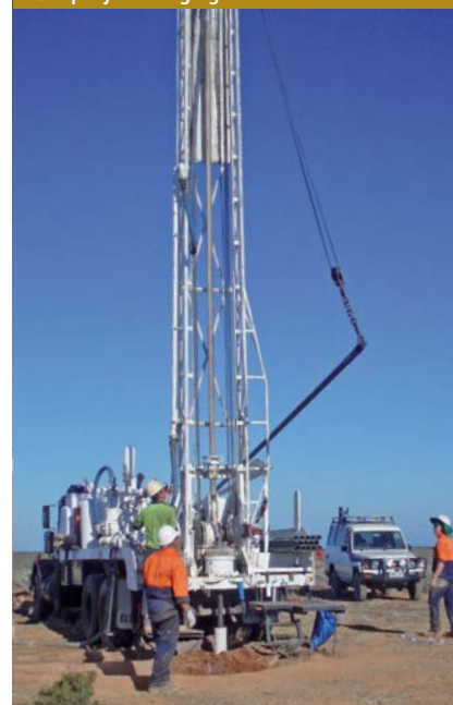
Company's drilling rig
